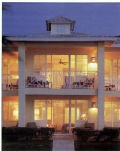
LEFT: One of nine plantation-style lodges, which contain varying numbers of individual rooms. The buildings have two or three stories, with five guest units on each floor.
